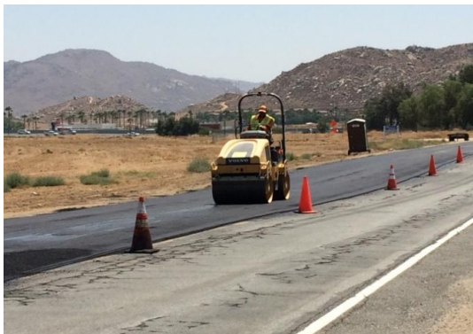
Pavement Rehabilitation Program
