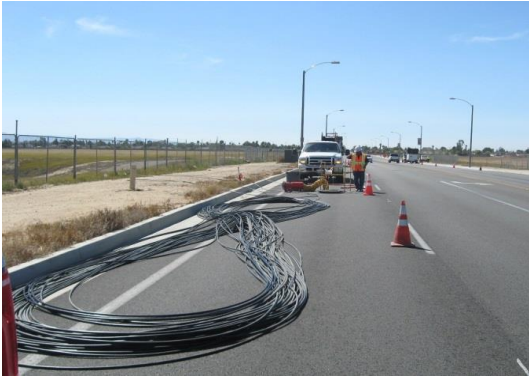
Citywide Fiber Optic Communications Expansion
