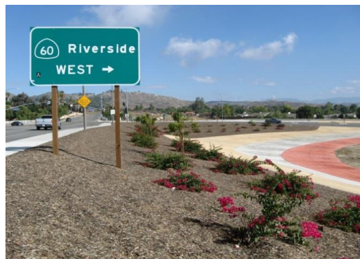
SR-60 / Nason Street Overcrossing Bridge (Landscape Establishment)
