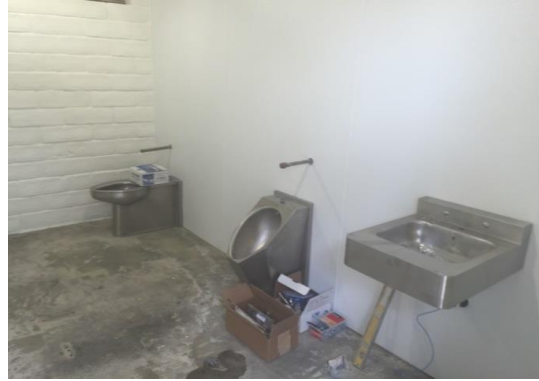
Park Restroom Renovations
