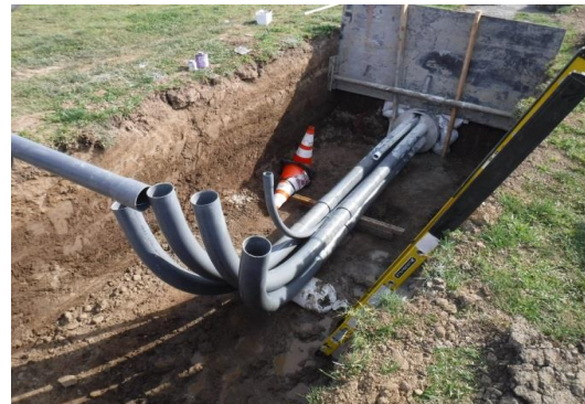
Feeder Line Trenching
