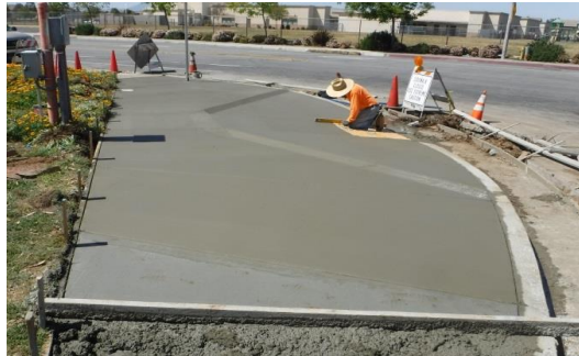
Pedestrian Ramp Improvements
