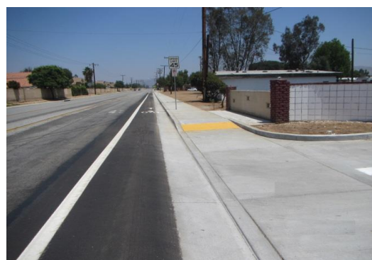
Pedestrian Ramp Improvements
