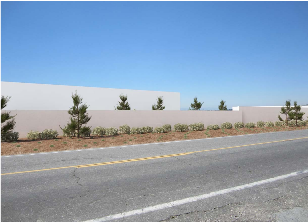
Gilman Springs Rd. View 5 at Installation
