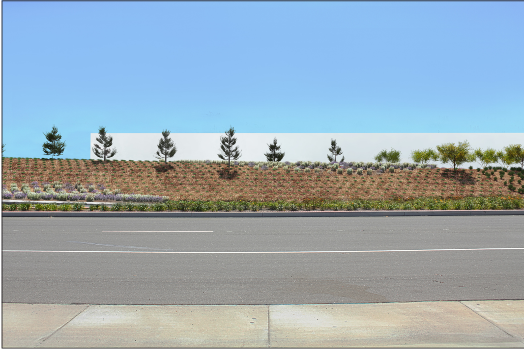
VIEW 1: View of Site 1 vegetation at installation.
