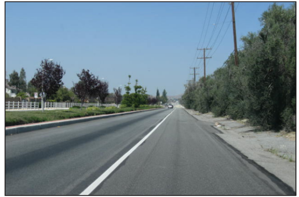
PHOTOGRAPH 2: View looking north along Redlands Boulevard from Alessandro Boulevard.
