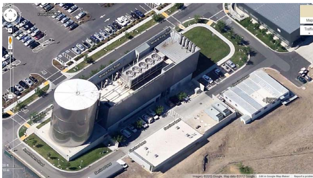
Chilled Water Storage
