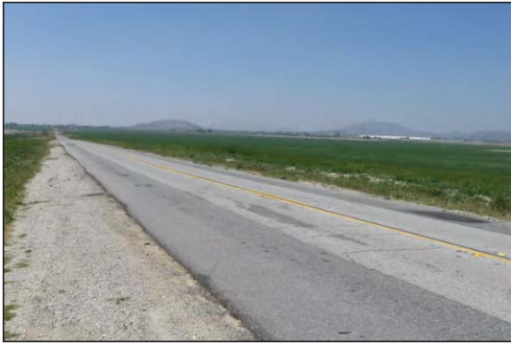
PHOTOGRAPH 11: View looking west along Alessandro Boulevard from near Gilman Springs Road.
