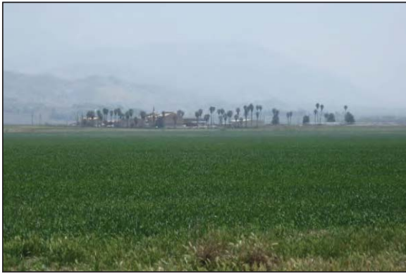
PHOTOGRAPH 7: View of SDG & E Natural Gas Compressor facility (central portion of site).
