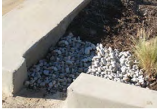
Figure 2: Curb Cut located in a Bioretention Facility
