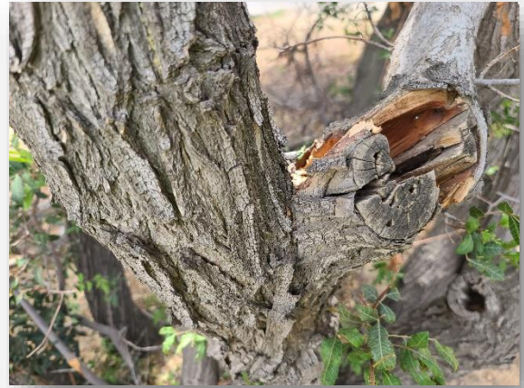
Plate 6. This is a view of bore holes within a branch cut (#365).
